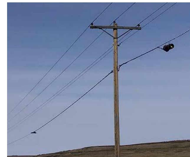
Fiber Aerial Slack Loop and Splice Case Application:
