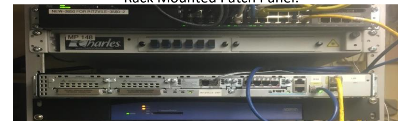
Rack Mounted Patch Panel:
